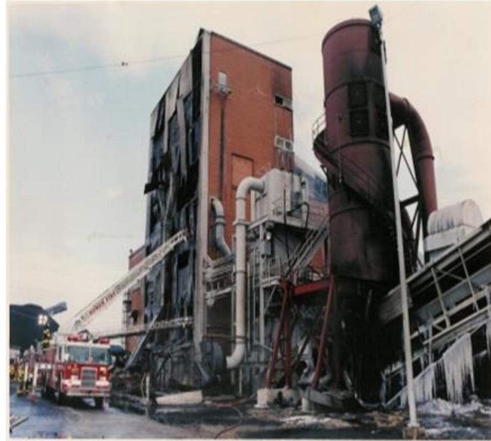
Will County Power Plant Crusher Building Explosion
