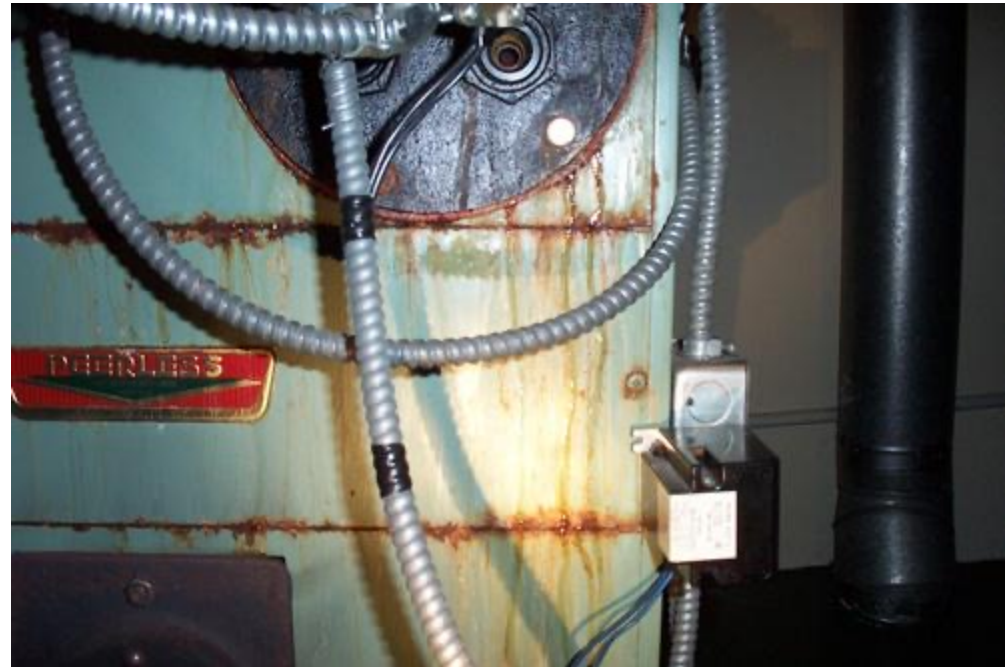
Boiler leak
