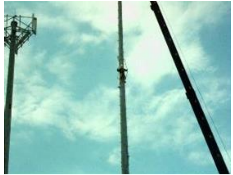
Ironworker using rope grabs to make tower connection.
