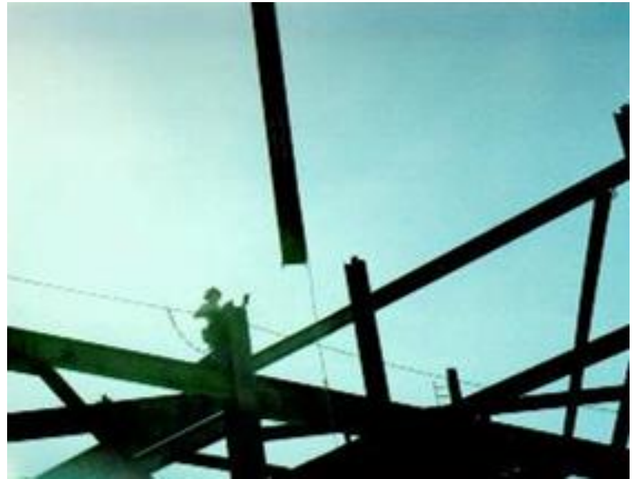
Perimeter cable system
