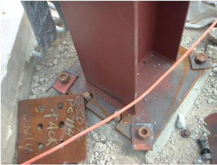
Four bolts used
